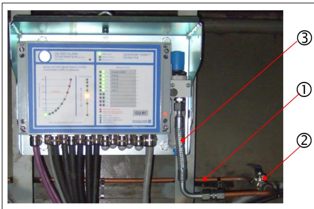
Fig.: 14 : Example of an optimum compressed air supply to the VN301 plus central unit
